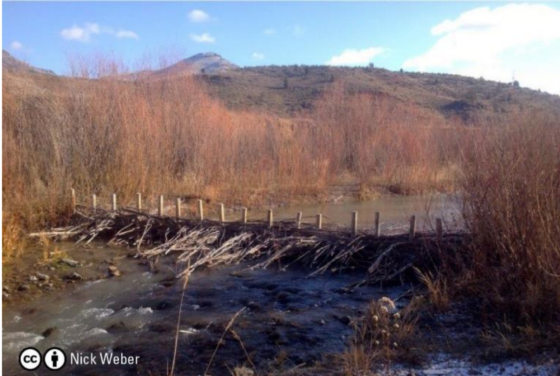
Figure 4: "Early generation BDA. The structure is characterized by a tight willow weave and limited downstream mattress, leaving it more susceptible to scour that can undermine the posts. The downstream mattress shown here was built by beaver, and provided the original inspiration for incorporating mattresses into BDAs which diffuses flows coming over the dam." (J.M. Wheaton, Bennett, Bouwes, Maestas, & Shahverdian, 2019)
